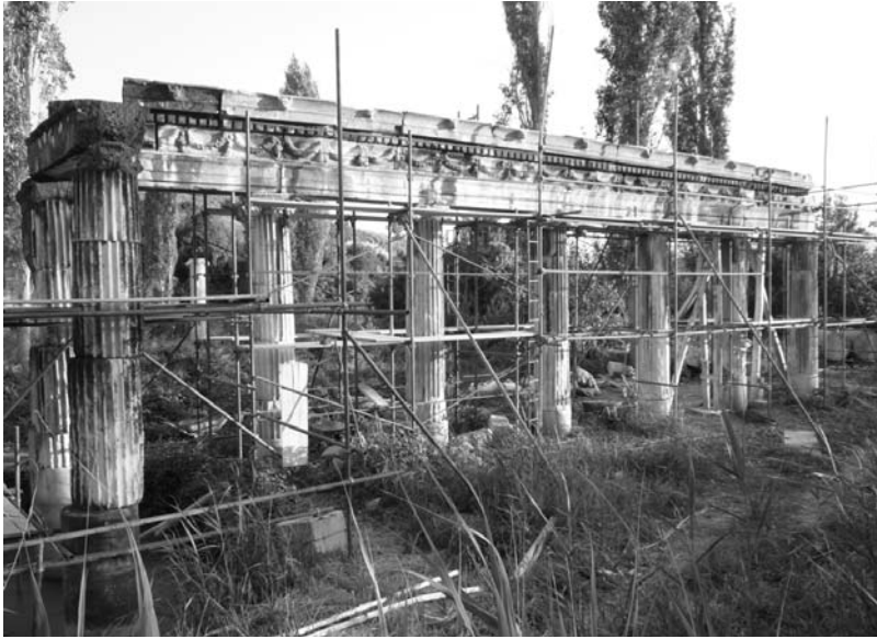
Above: the colonnade of the North Agora's South Stoa under scaffolding for repair work and cleaning. Fine water sprays were played over the blackened surface to soften the deposits of centuries of town and village smoke. Right: work to stabilise a seriously damaged column.
