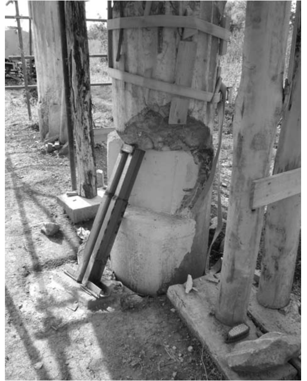
Above: the colonnade of the North Agora's South Stoa under scaffolding for repair work and cleaning. Fine water sprays were played over the blackened surface to soften the deposits of centuries of town and village smoke. Right: work to stabilise a seriously damaged column.
