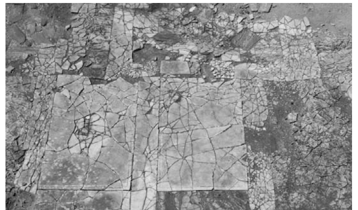
Left: prior to any treatment, a trial area of shattered marble floor is cleaned with a vacuum cleaner – a sieve prevents the marble from being removed in the process.
