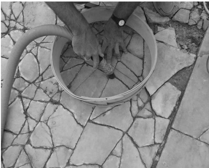
Left: prior to any treatment, a trial area of shattered marble floor is cleaned with a vacuum cleaner – a sieve prevents the marble from being removed in the process.
