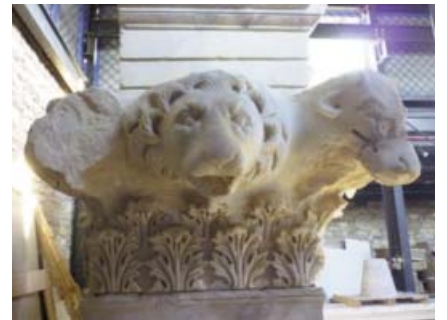
Composite pier capital from the South Hall of the Civil Basilica with newly-identified and restored bull's head from the depot.
