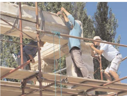
Repairing columns and piers of the Sebasteion Propylon in the conservation workshop.
