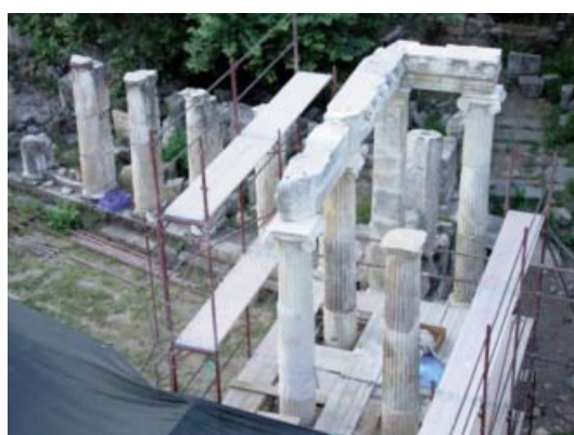
The Sebasteion Propylon during the 2014 season: anastylosis of its Ionic columns and architrave friezes.
