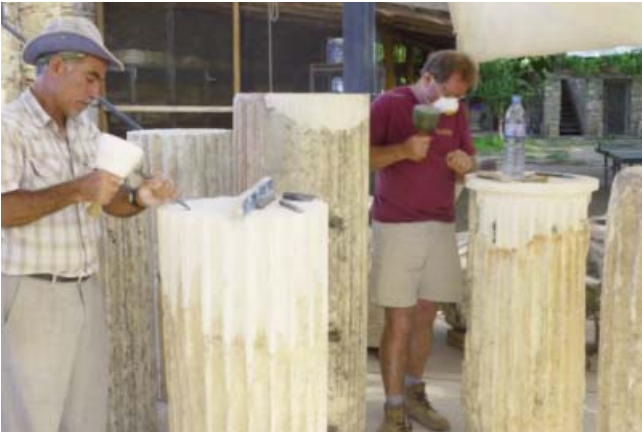
Repairing columns and piers of the Sebasteion Propylon in the conservation workshop.
