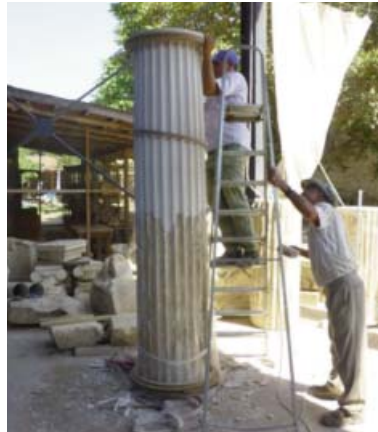
Repairing columns and piers of the Sebasteion Propylon in the conservation workshop.
